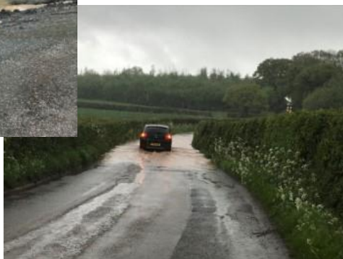
White Cross Road Woodbury Salterton Surface water flowing off field. There is a ditch on the field side of the hedge is could go into.
